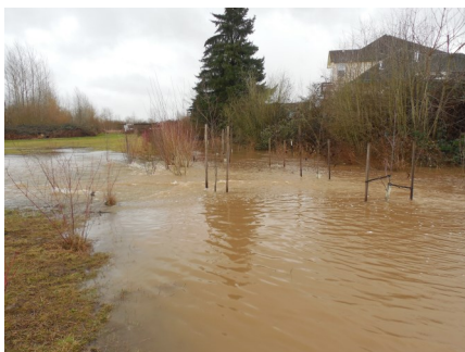
Labish Creek during a high water event in the winter of 2017 spills it's banks at Country Glen Park.
