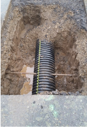
A "cross bore" of a natural gas line through a storm line is a common occurrence since Horizontal Directional drilling (HDD) became a routine way to install underground utilities.
