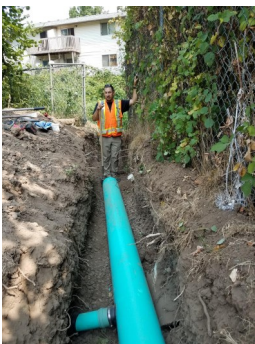
Greg Hamilton lays some storm pipe on the Faymar Ave. outfall repair this summer.
